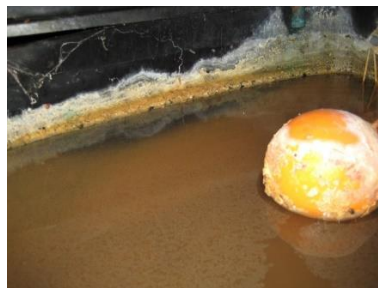
Uncovered storage tank
